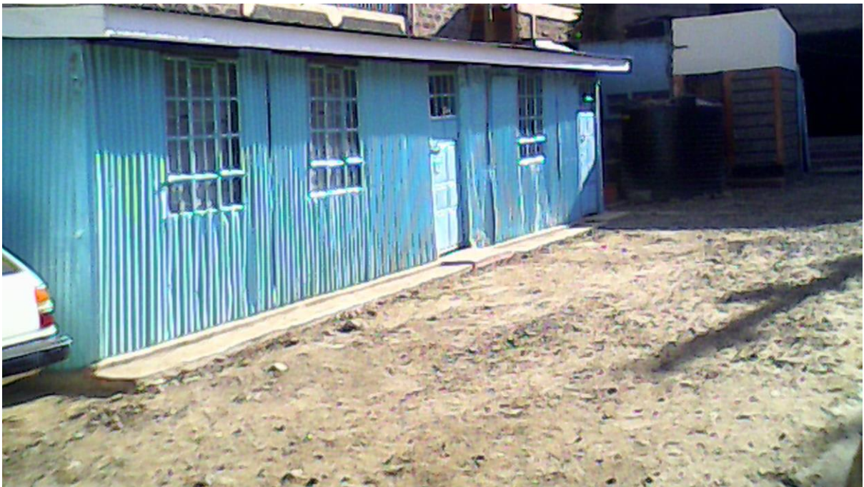
The two mabati classes for Sunday school were constructed during this time, and the Vicar's Toilet can be seen attached to the old toilets at the background.
