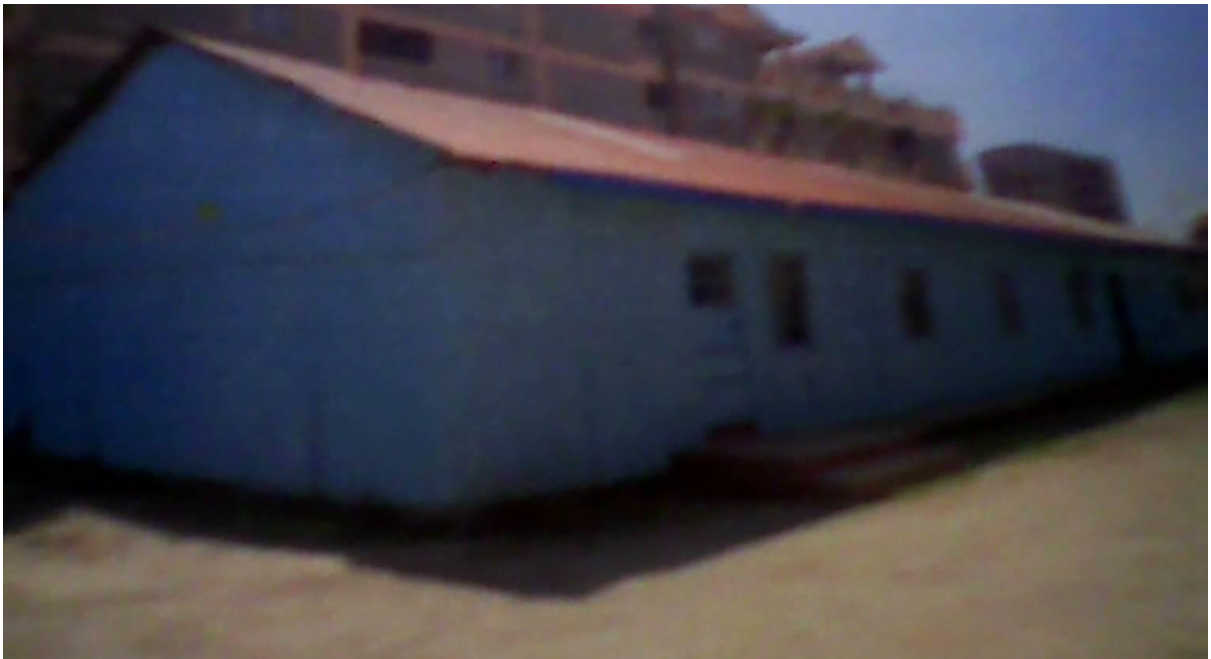
The Church seen after the extension. The church could now house over five hundred congregation.
